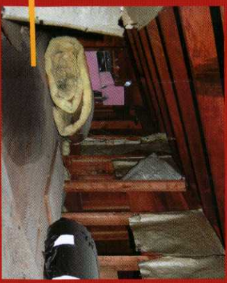
■ Leakage in attic after driving rain. Possible causes: Leaky or inadequate shingle underlayment; deteriorated flashing.
