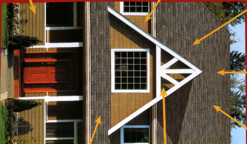
■ Leakage in attic after driving rain. Possible causes: Leaky or inadequate shingle underlayment; deteriorated flashing.
