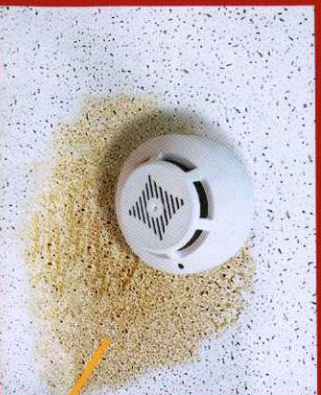
■ Stains on interior ceilings and walls or mold and mildew growth. Possible cause: Inadequate or faulty shingle underlayment allowing leakage, or inadequate ventilation.
