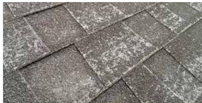
SBS provides better adhesion to hold the surface granules better and allows the shingles to endure extreme weather longer.
