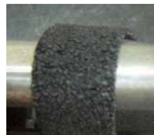
SBS - modified asphalt shingle with no cracking
