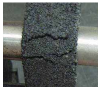
non-modified asphalt shingle with cracking
